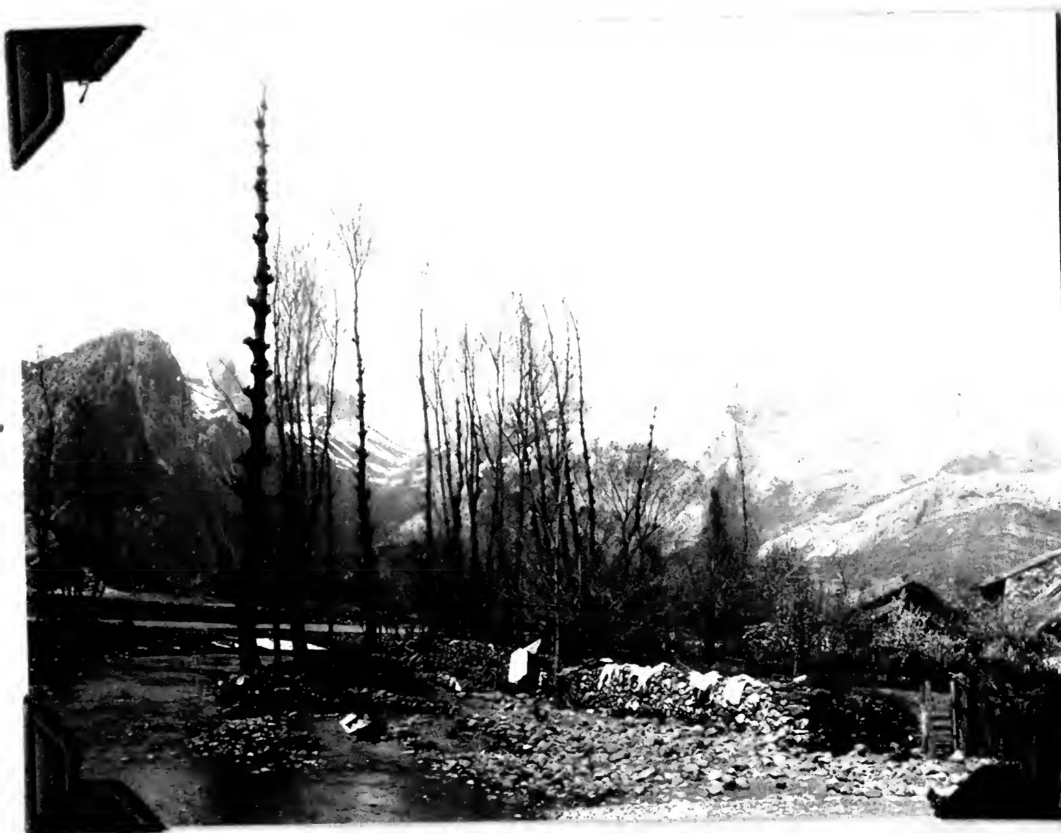
2009. A channel of the Río Esla in the outskirts of Riaño. May 13, 1930.
